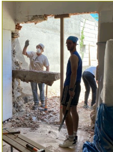
Right: Making the connection. The Pitman group helped install a new door connecting the church to the new Leydet Property (see photo below).
