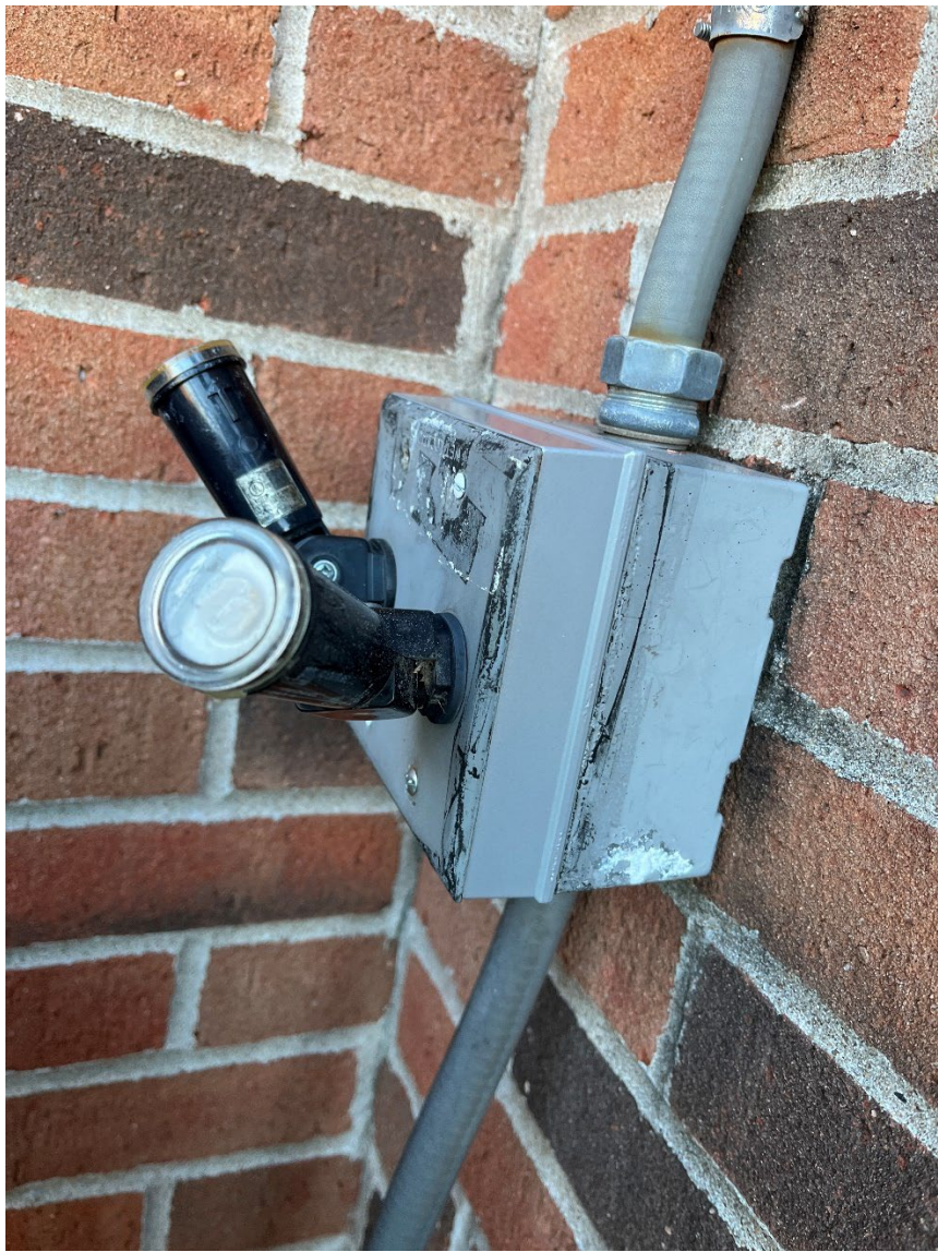
I added an extension to the 2-gauge exterior box
